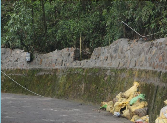
Construction of protection Wall
