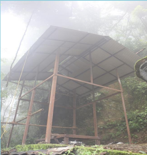
Renovation of Animal carcass burning shed
