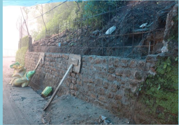
Maintenance of Wall /Fence
